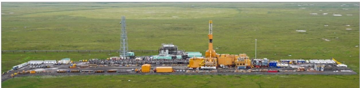
Figure 21. Example of infrastructure and pipelines in the GMT-2 area.
